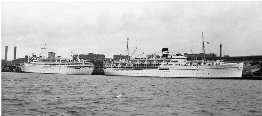
The stage could accommodate two liners (Devonia and Aureol) shown in the picture) and raised access gangways were provided for passengers. The floating roadway allowed vehicular traffic for baggage and stores. Riverside station could take main-line trains with passengers having easy access to the ships.
